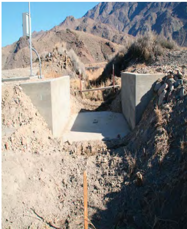
Concrete Box Weir
